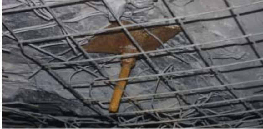
Figure 26: Damage to bolt head due to blasting at Doyon Mine
