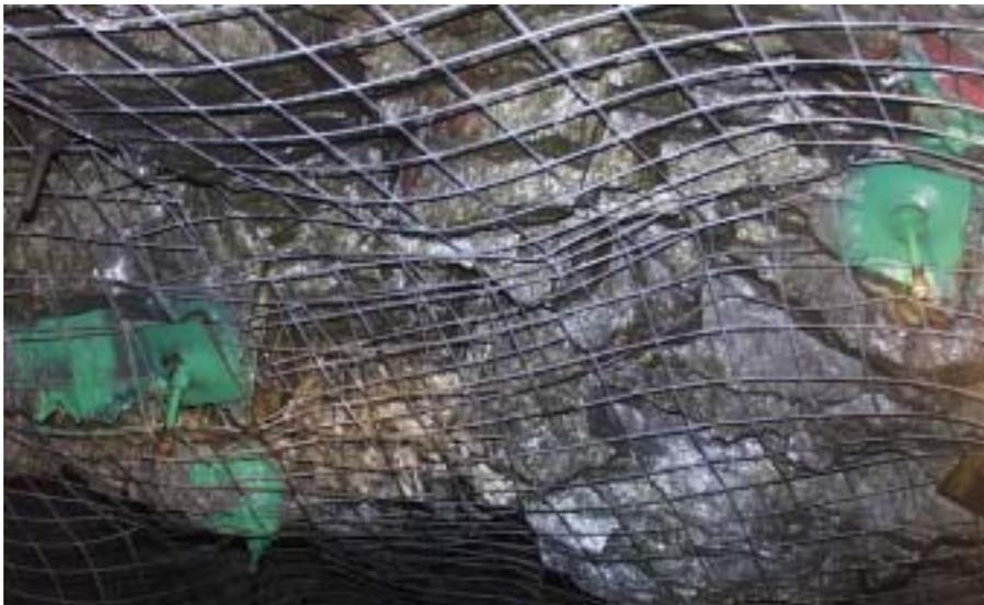
Figure 24: Identification of instrumented bolts using spray paint
