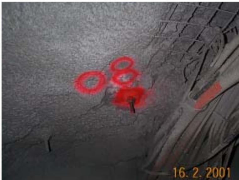
Figure 42: SAFEbolt-instrumented bolt No.8
